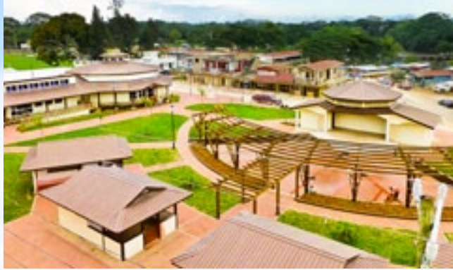
The construction of the new visitor Welcome Center in San Ignacio / Cayo was completed in 2012.
