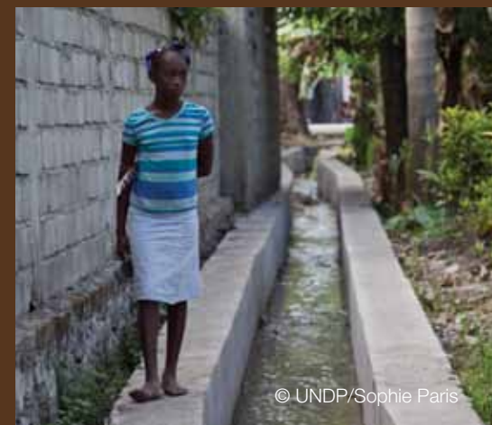
Cleaned channel, les Cayes
